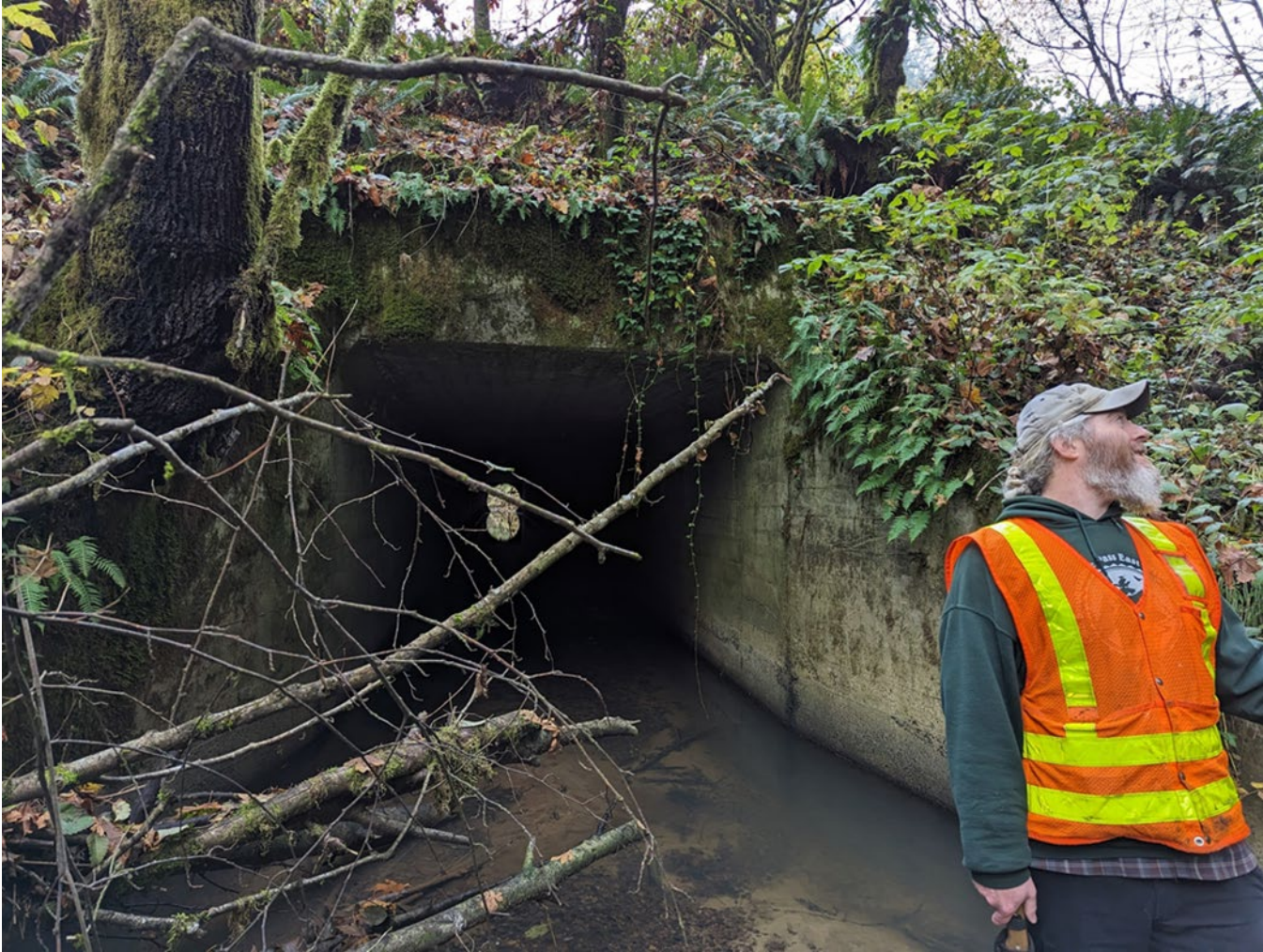
Figure 5-10. MP 56.1 UNT Hill Creek culvert inlet during November 2023 site assessment.
