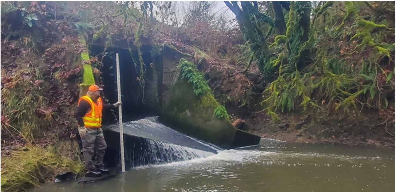
Figure 5-13. MP 58.6 Foster Creek culvert outlet from December 2023 WSDOT fish passage assessment.
