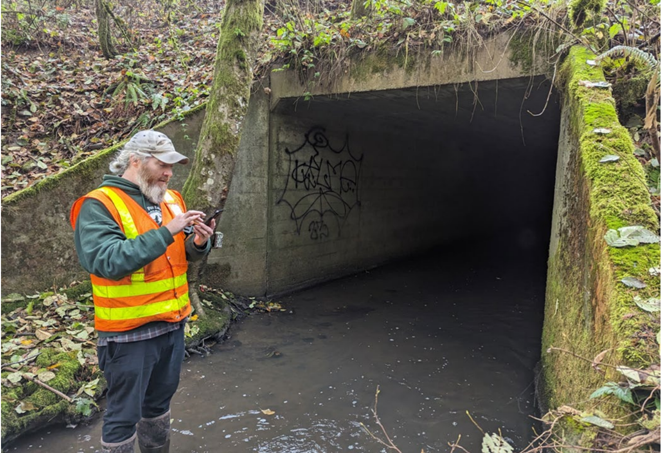
Figure 5-12. MP 58.6 Foster Creek culvert inlet from November 2023 site assessment.
