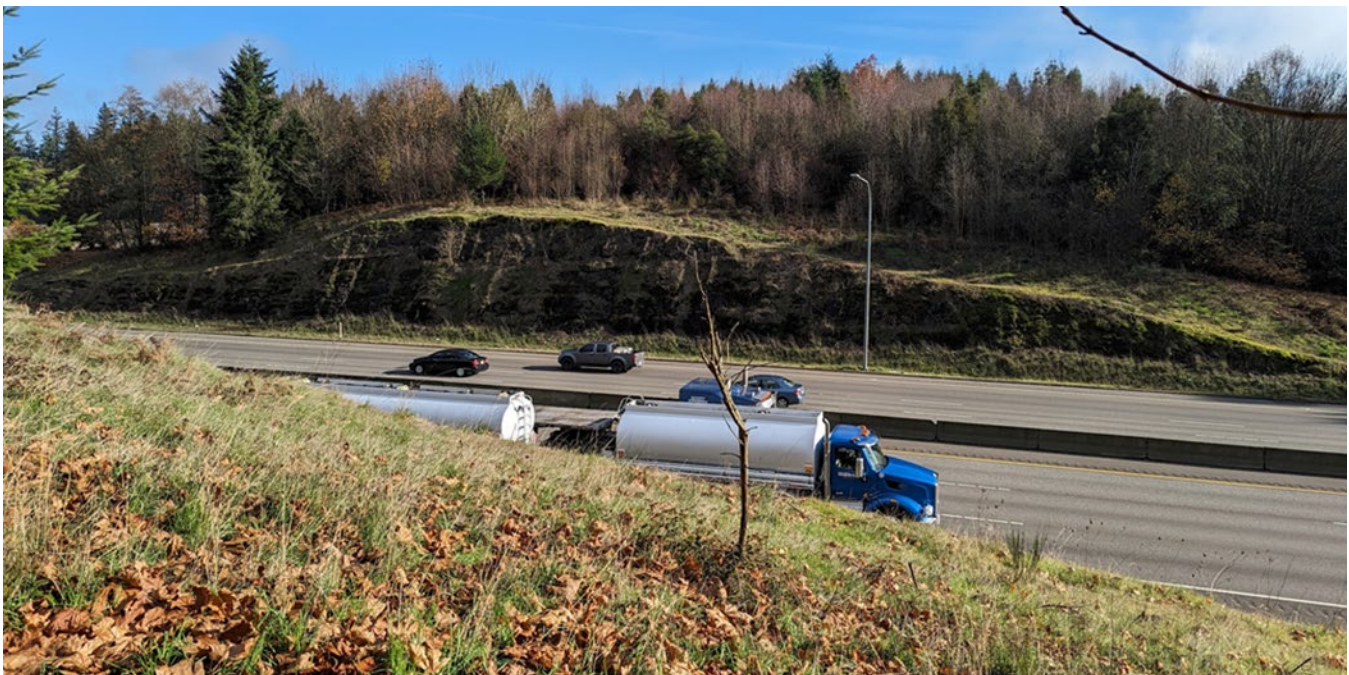
Figure 5-19. The top of the basalt roadcut at MP 96.1 is approximately 40 ft above the existing road surface. Photo taken from west side of highway looking east during November 2023 site assessment.
